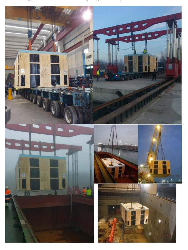
Door to door delivery of 1 x Exchanger (22 meters long and weighting 121 tons) from Cremona to Grangemouth including road transportation up to Porto Marghera, loading onto vessel, sea transportation from Porto Marghera to Grangemouth port, discharging and road delivery up to job site (Final Client: INEOS Plant).
