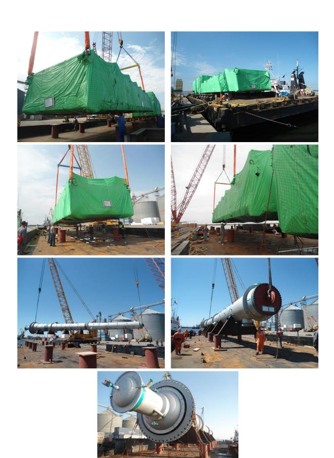
Road transport from Manufacturer up to Porto Marghera, loading and ocean transport up to Paranagua (Brazil) of 1 Steam Drum measuring 19 x 3.5 x 4.5 and weighting 201 tons – UFN III Plant (Petrobras).
