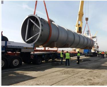
Sea transportation by ro/ro barge of 1 x Column (measuring 51 x 7 x 7 meters and weighting 255 tons) from Ortona port to Rijeka, Croatia (Final Client: INA Refinery).
