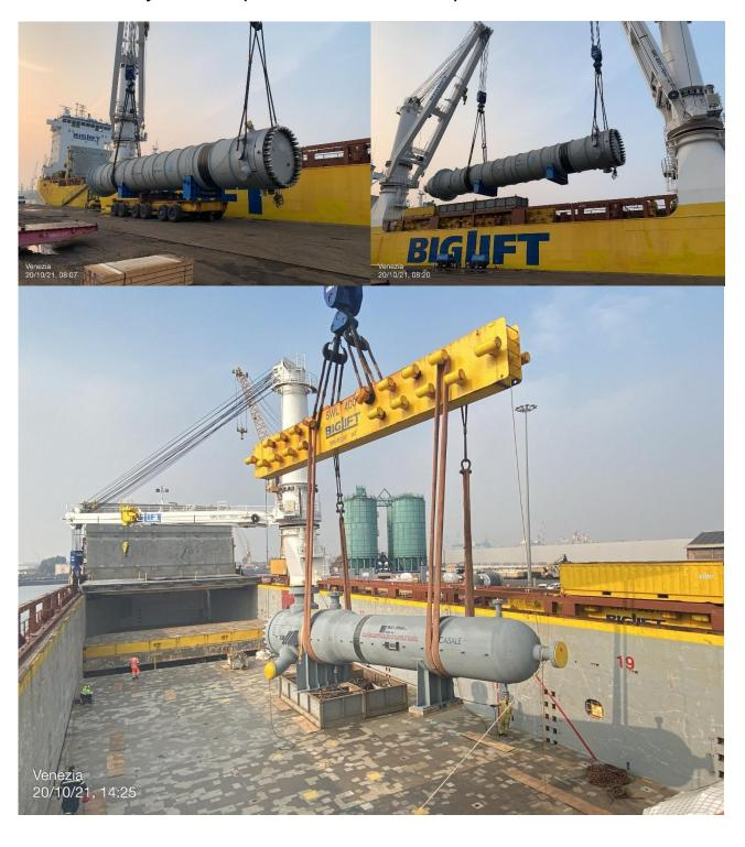
Ocean transportation from Ortona to Rayong port, discharging and road delivery up to job site of 1 Reactor measuring 23.0  $\times$  6.6  $\times$  5.3 m and weighting 178 tons (Final Client: IRPC Plant).
