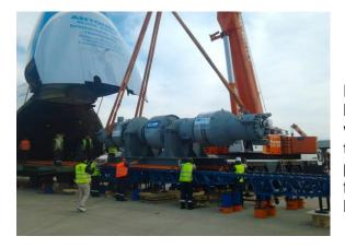
Loading operations of the Stripper and the Reactor have started at 3.30pm. 3x200t jib cranes have been working as a whole to load and position the items on the ramp with the utmost caution and accuracy. The plane winches have allowed the sliding of the items from the ramp to the final positioning into the AN-225 hold.
